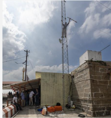
OM Deepan installing the wire 3 antenna
