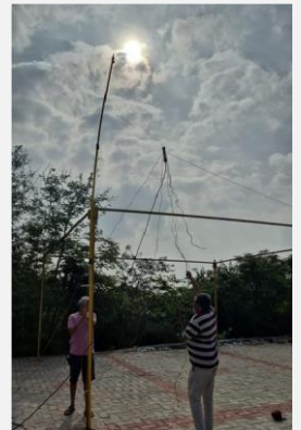
Hoisting the dipole
