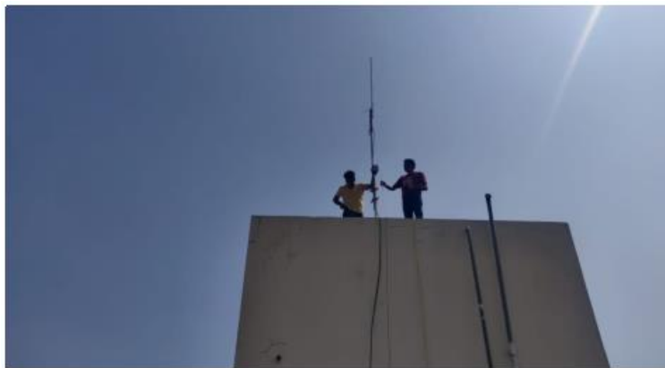
VU3UBN and VU3OIM going atop the water tank above the terrace and installing the X50 VHF/UHF antenna.
