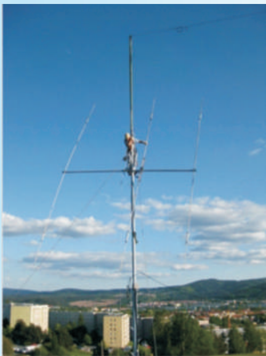
Andre fixing a 3-el Yagi at 20m
