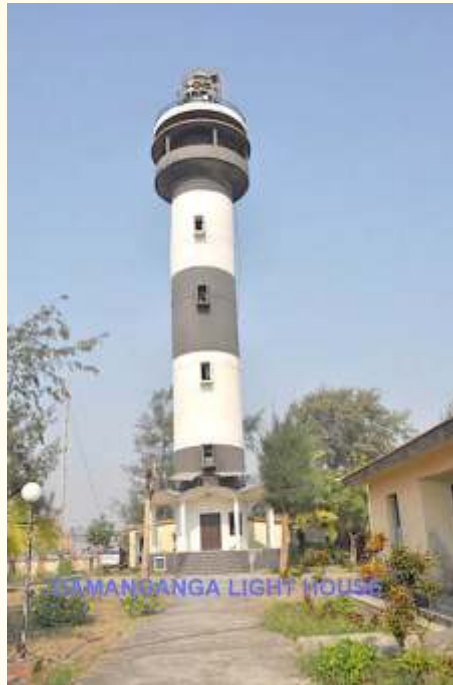
The Lighthouses are located in the Union territory of Daman, in Gujarat, grid location ML60jj.
